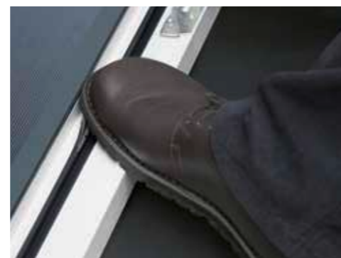
Centre gasket glued to the frame profile
