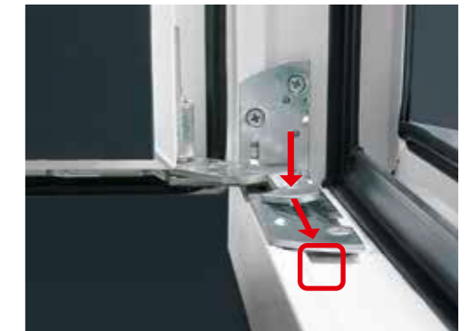
Corner hinge not fixed flush in frame
